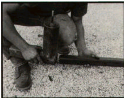
17 Depending on your application, during assembly use 3/8" three-inch long bolts with nuts and try and get the center round rotating stock to a height that would be in the center of your body or frame. This will promote easiest rotating. Slide the adjustment slider #9 onto the main standing support #1.
